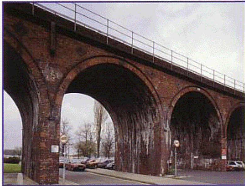
Worcester Viaduct, England
