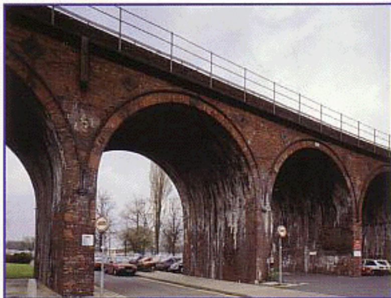
Worcester Viaduct, England
